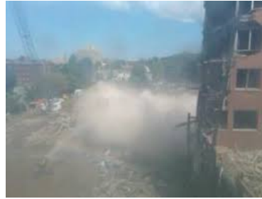
demolition of Genesee Hospital
